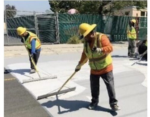
Reflective or “high albedo” pavements include light-colored roads, sidewalks and parking lots. These pavements use a reflective sealant to bounce sunlight and heat away from cities to reduce surface temperatures.
