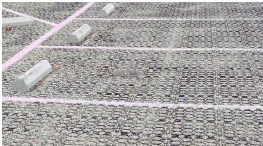
Porous pavements allow rain to pass through the surface, recharging groundwater while reducing flood risk.
